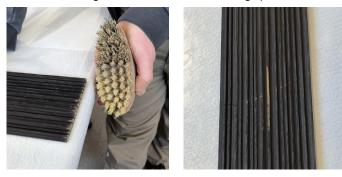
2. Apply a thin layer of Touch-Up Ridgeline to the damaged areas with a fine brush and remove excess with a disposable paper towel.
